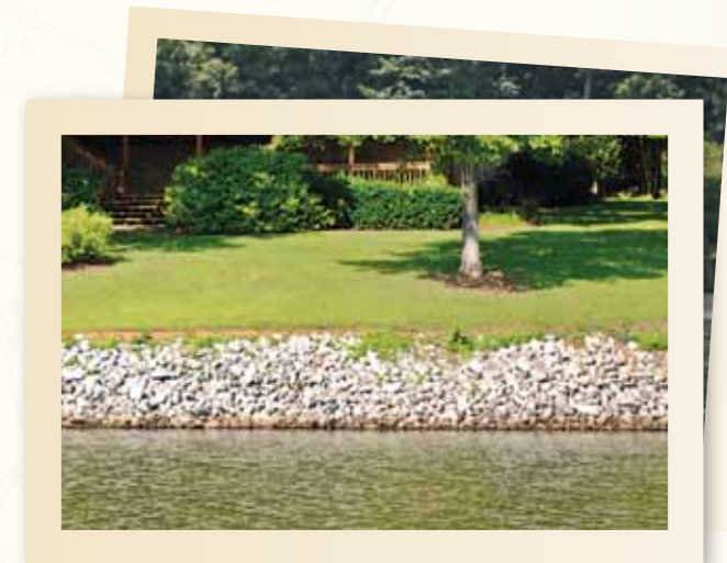
Riprap is the sloped piling of rocks 4-6 inches in diameter and is recommended for most shoreline stabilization projects.
