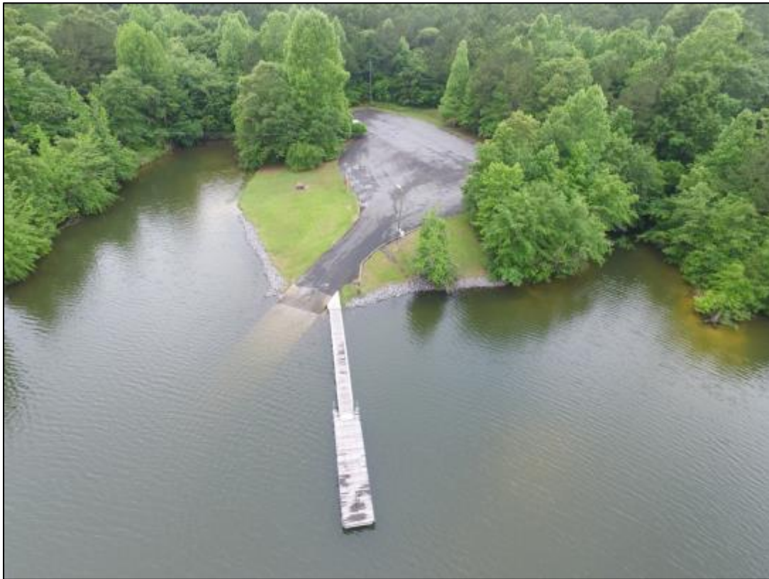
Boat Ramp and Barrier-free Launching Pier
